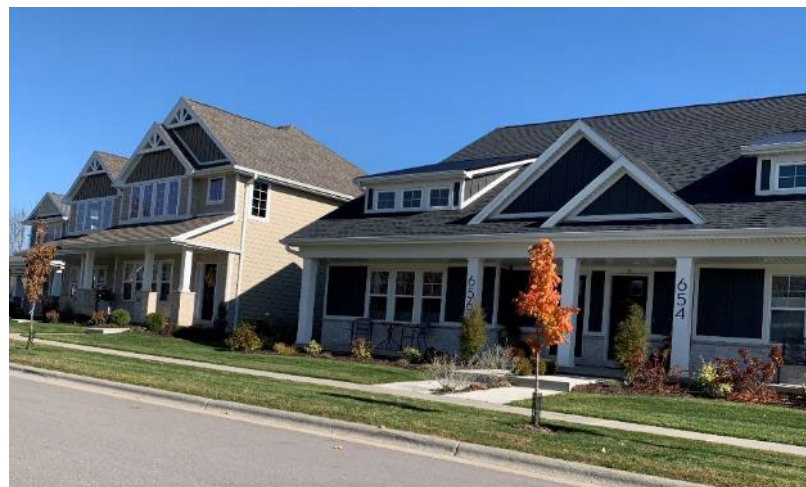
This complete neighborhood example from another community seamlessly blends duplexes with single-family homes.
